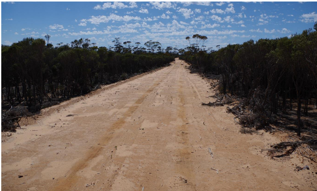
Plate 11: Example of topographic valley crossings the haul road area
